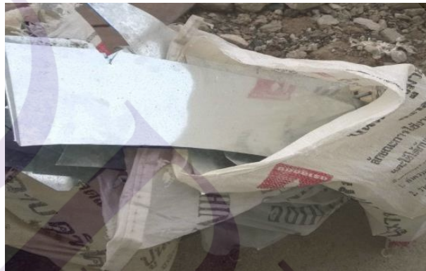
Material and Waste Management / location of material and Waste on site
