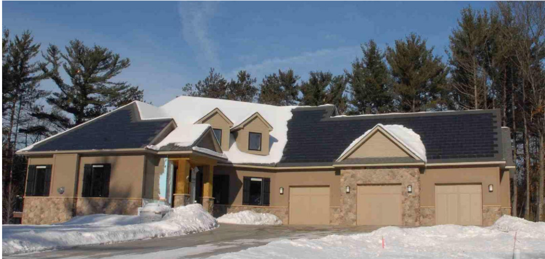
FIGURE 14.4 A pilot project of the BITER system.
