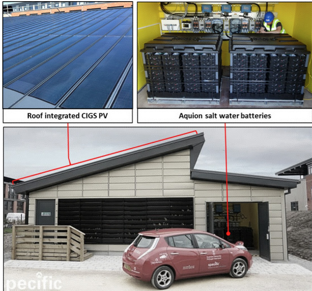
FIGURE 5.1 The SPECIFIC 'Active Classroom' with roof integrated PV and salt water batteries.
