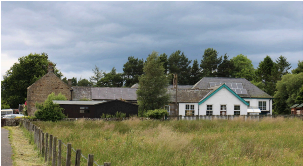
FIGURE 19.2 Solar panels retrofitted onto existing buildings, Otterburn First School, Northumberland UK. Photo: B. Dower (all rights reserved).
