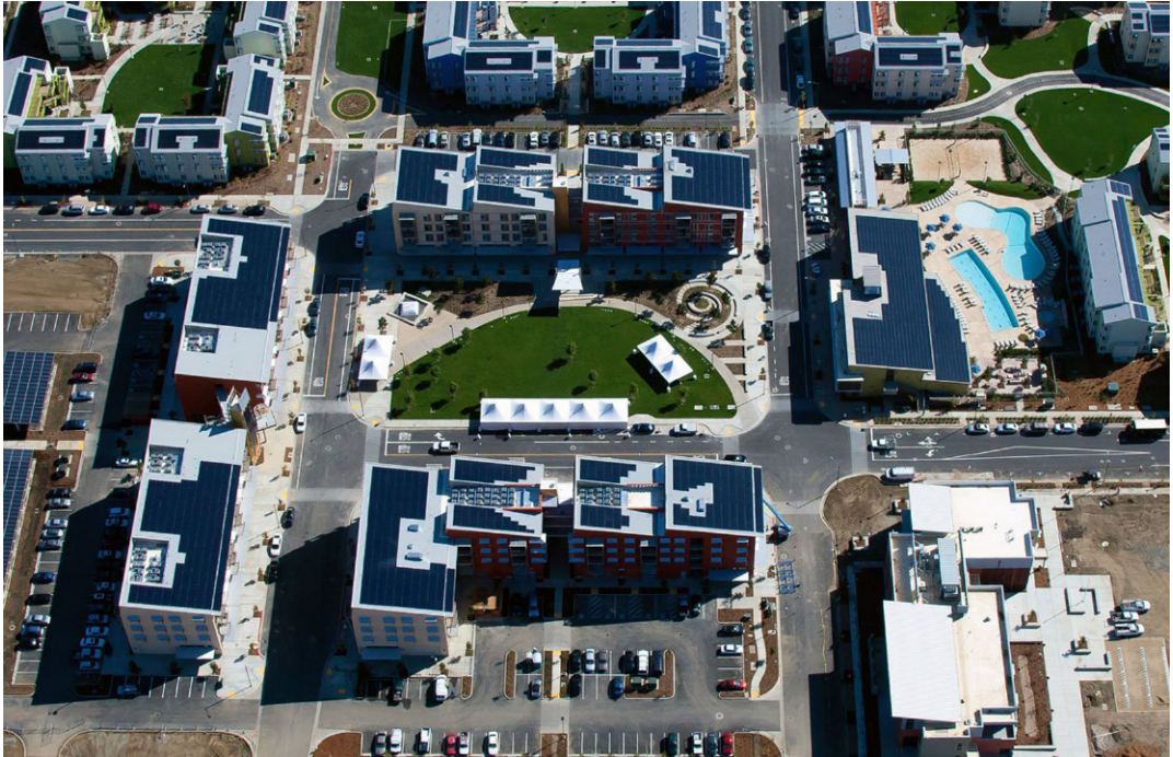
FIGURE 20.2 Aerial view of 4.1 MW of integrated solar energy at the UC Davis West Village. West Village is the largest net zero energy community in the United States, combining energy efficient technology with on-site energy production via rooftop and vertical photovoltaic installations (Davis, California). Photo courtesy of UC Davis.
